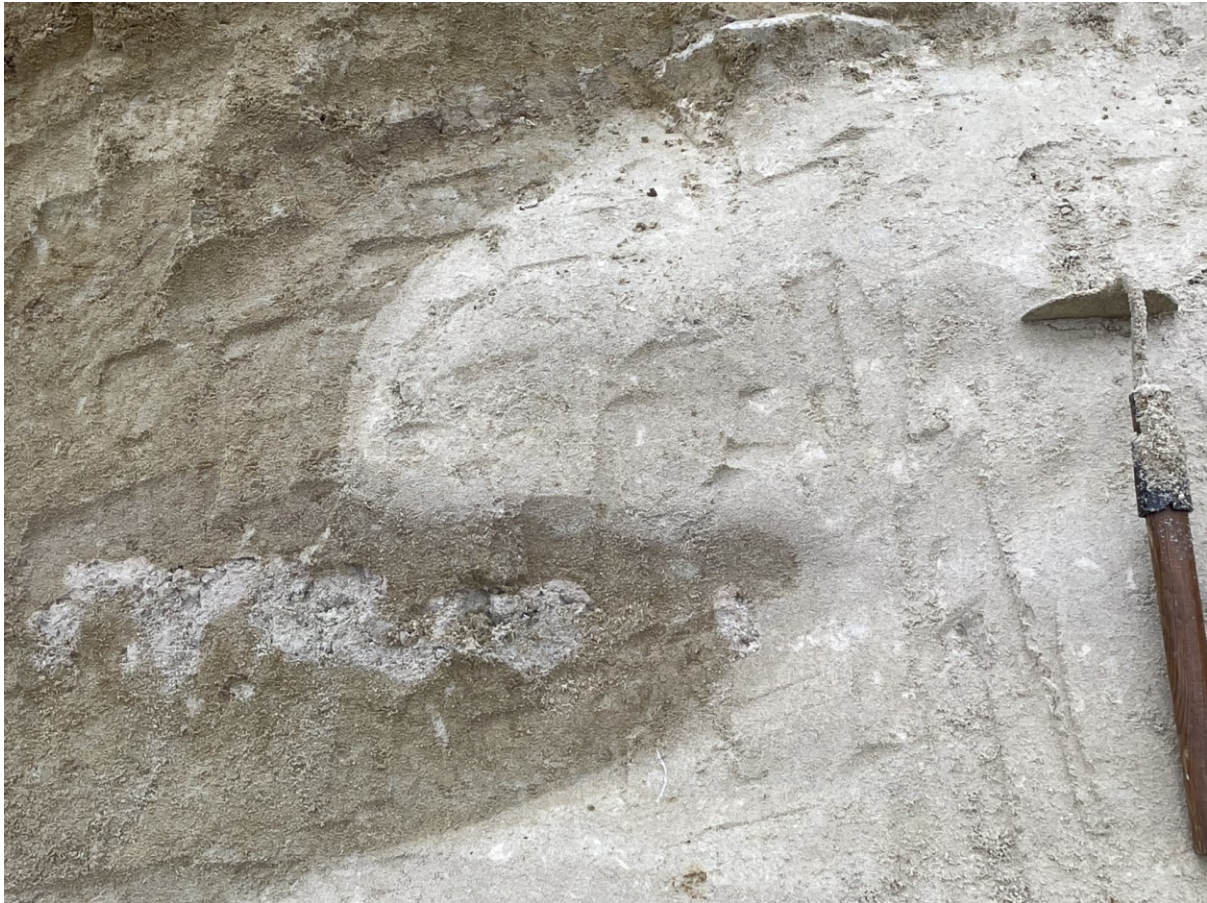
Calcareous (lower right) and decalcified (upper left) facies of the Machelen Member. Note sharp and capricious shape of interface surface.. Note disintegrated carbonate sandstone in middle of photo. Construction site in Diegem, 16/02/2022. Tool is 40 cm long.
